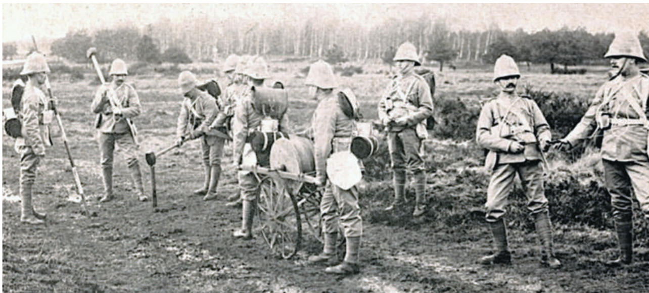
Figure 7: British sappers laying lines in South Africa.
