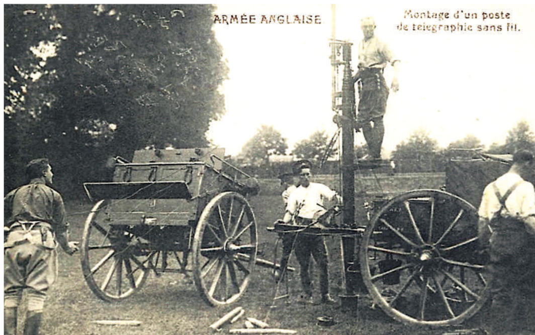
Figure 11: A telegraph communications post being installed "somewhere in France."
